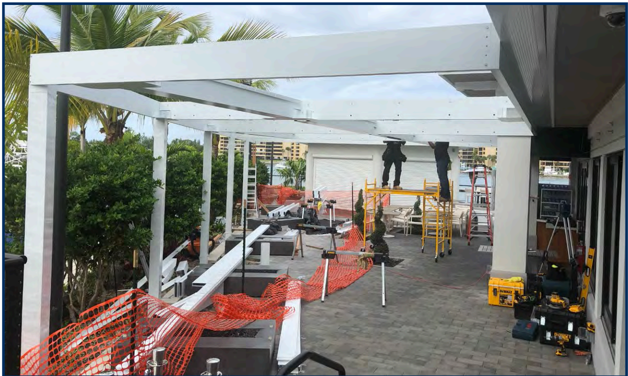
During Pergola Construction
