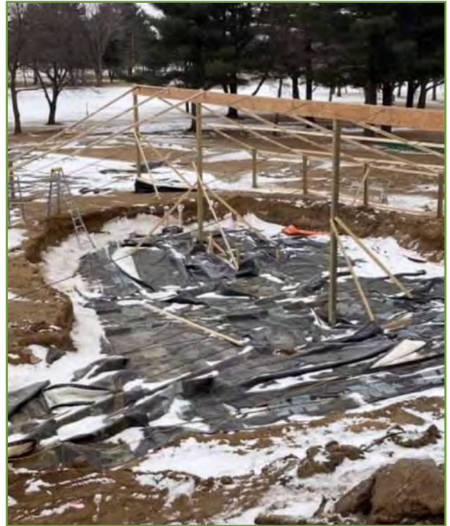
Zero Entry Being Prepared for Winter Construction
