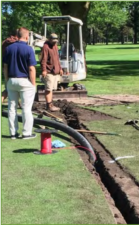
Course Drainage Work on 6 Holes – Added Fairway Drainage and Catch Basins in Rough
