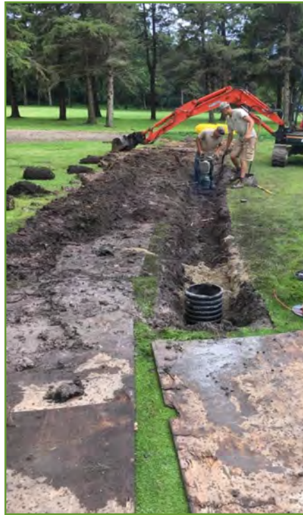
Course Drainage Work on 6 Holes – Added Fairway Drainage and Catch Basins in Rough
