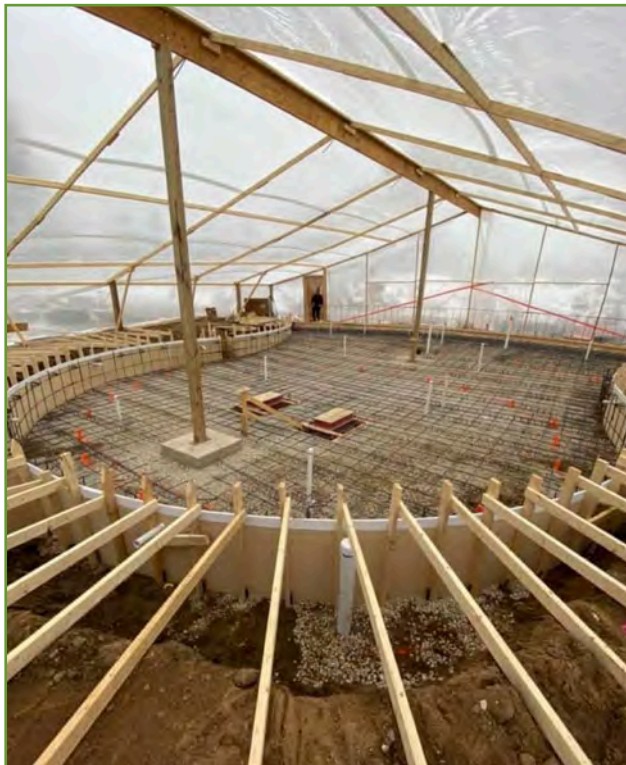
Formed & Ready for Shockcrete
