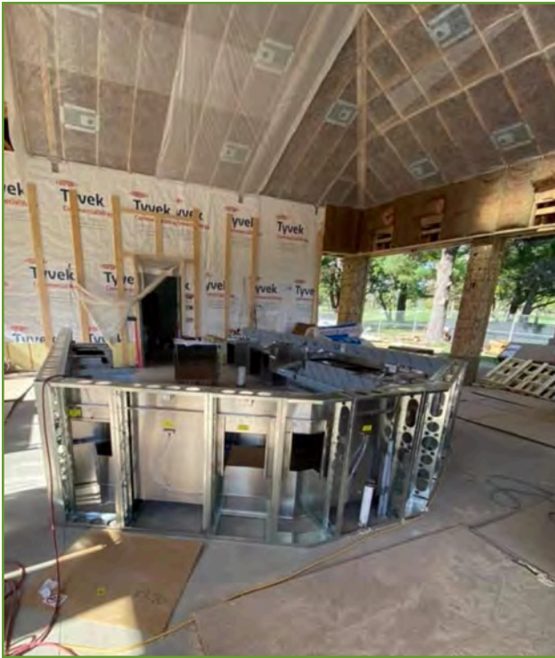
Cabana Slab Poured and Bar Die Wall Installed
