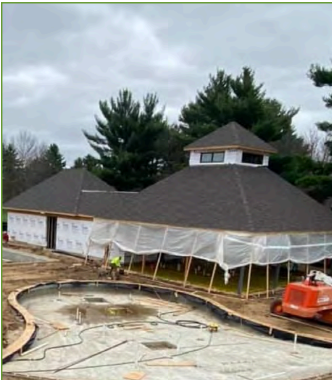
Cabana View from Upper Patio, Preparing to Pour Slab
