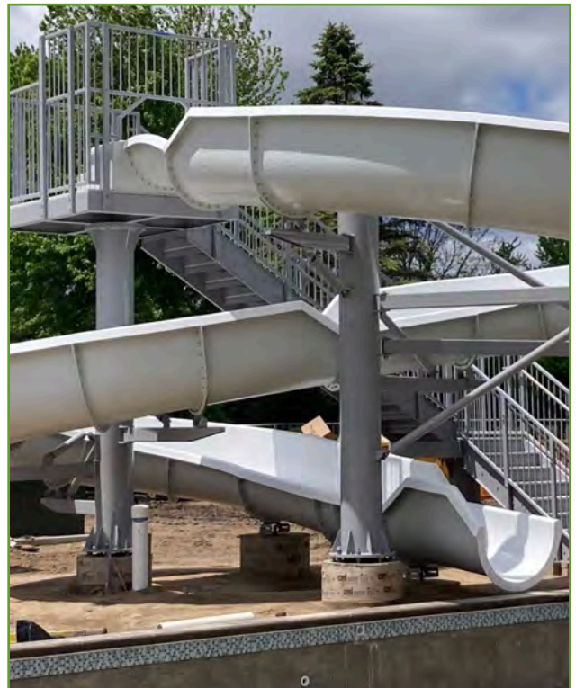
Slide Almost Completed
