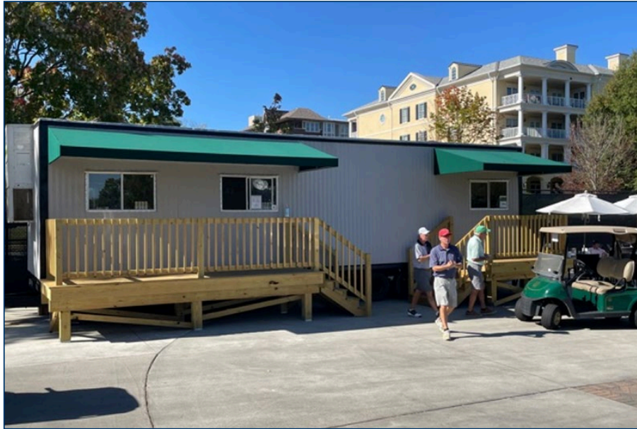
Created a Member Bar Trailer for additional beverage service at the golf facility while the club is under construction.
