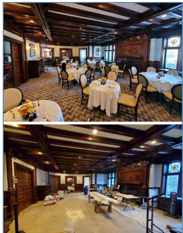
Private Dining Renovation
