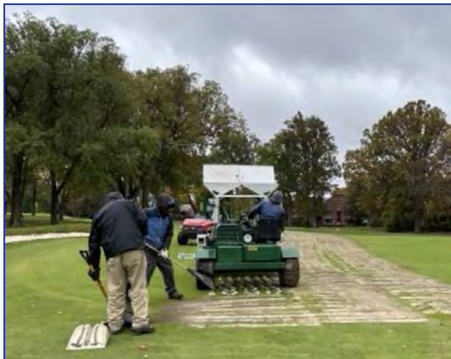
Drill & Fill Process
