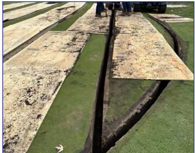
XGD Drainage System Installation
